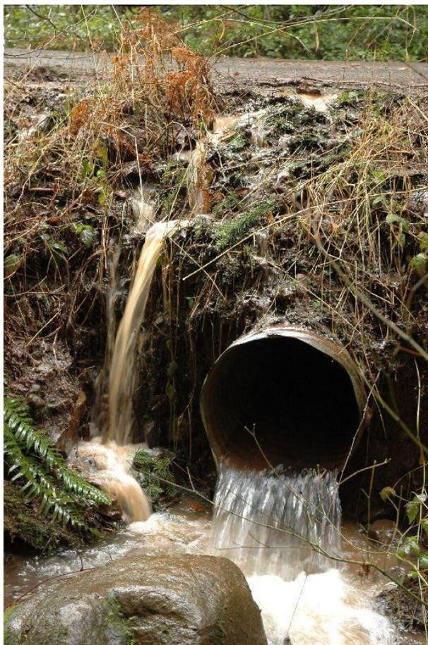
Runoff from Rd4610 drains directly into tributary of North Fork Clackamas River.
